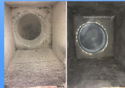
DHS Air Duct Cleaning
