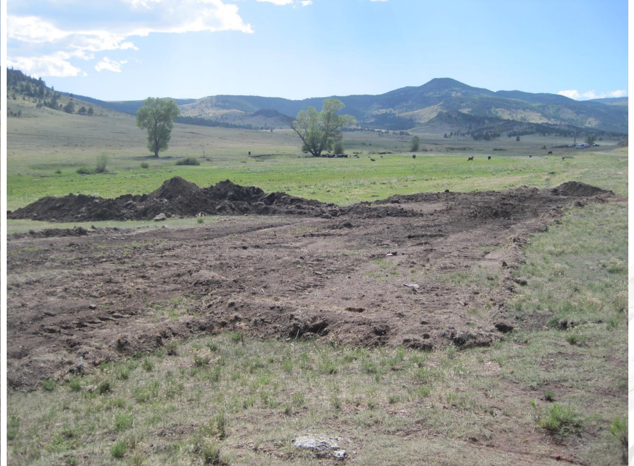
Drill pad excavated and topsoil stockpiled
