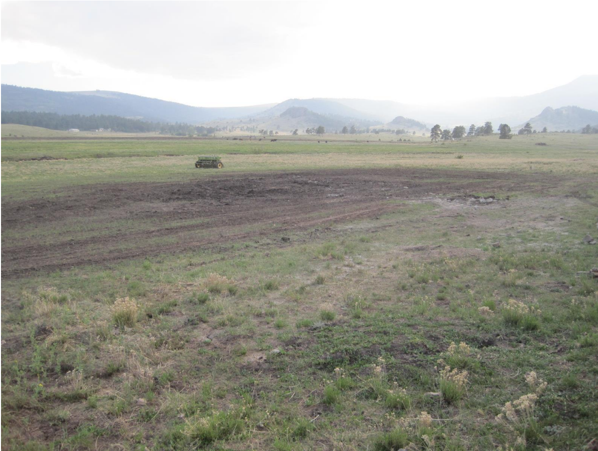
Drill pad reclaimed, raked and seeded
