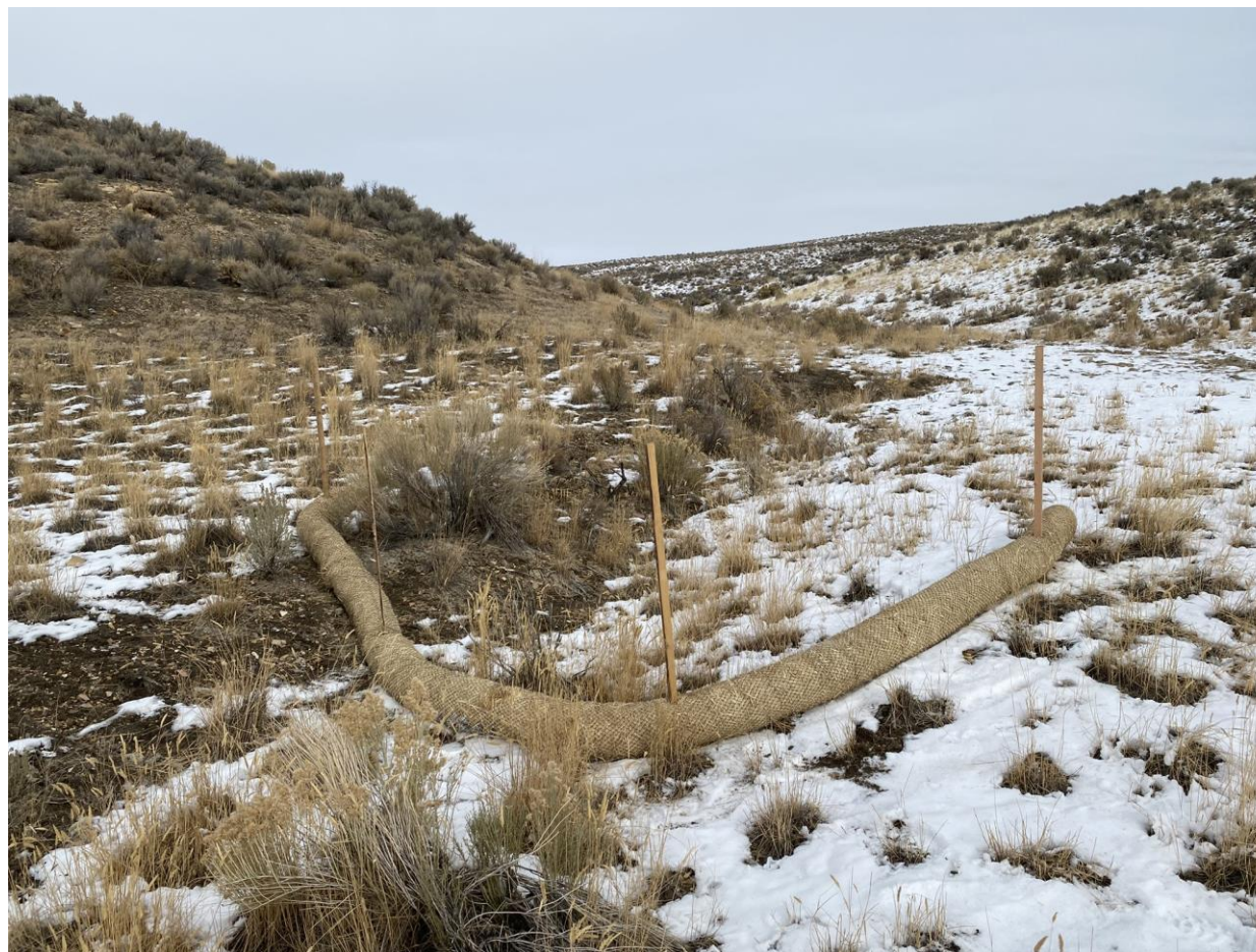
Wattles used to control sediment run-off
