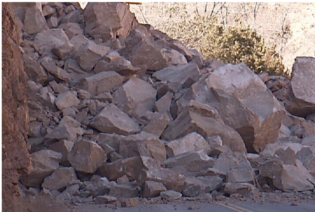
Figure 12-5. Cotopaxi Rockfall on Highway 50 in 2011
