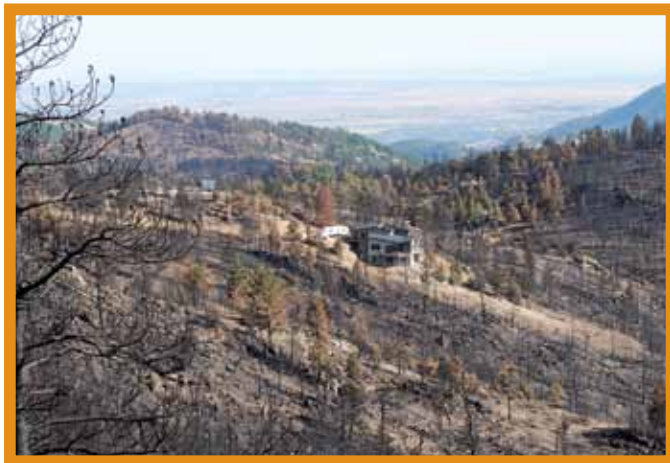
Figure 29: This house survived the Fourmile Canyon Fire in 2010. Photo: CSFS
