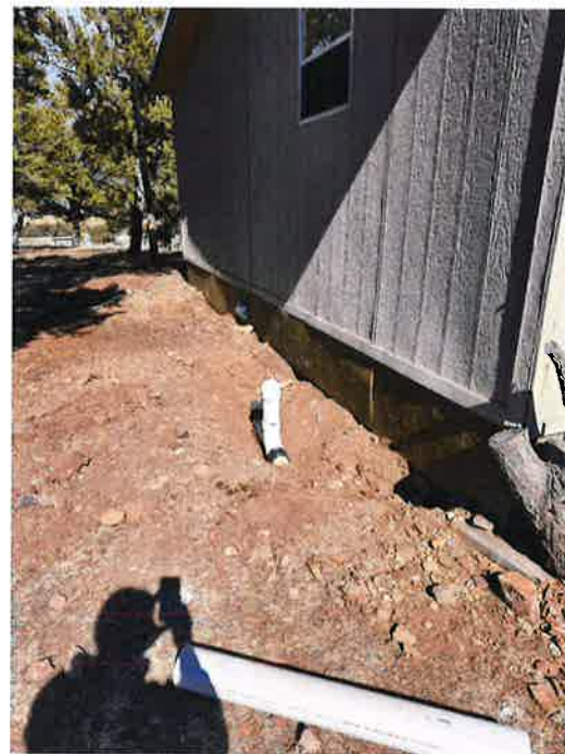
Newly installed 4" PVC clean-out of the west side of the home.
