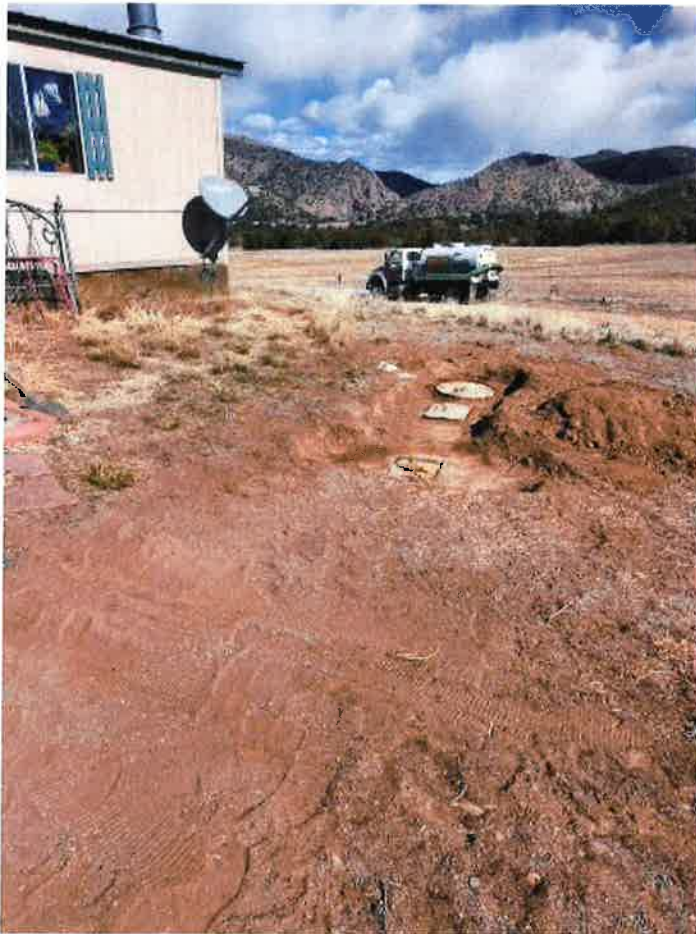
View of septic tank location on the south side of the home.
