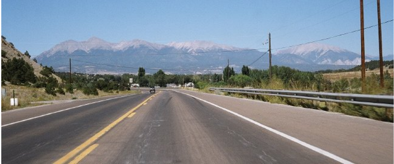
U.S. Highway 50 looking westerly near the Fremont-Chaffee County line.
