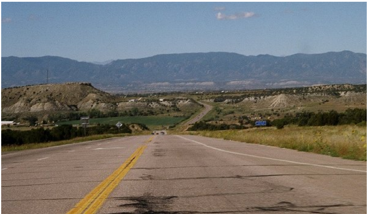
C.S. Highway 115 looking southerly as it approaches Penrose.
