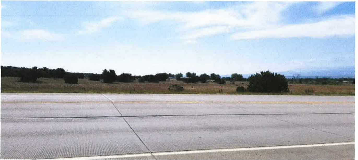
Continuing southbound still looking across at site location.
